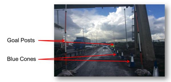
GS6 is there to indicate a structure or overhead power line is in your work area.
